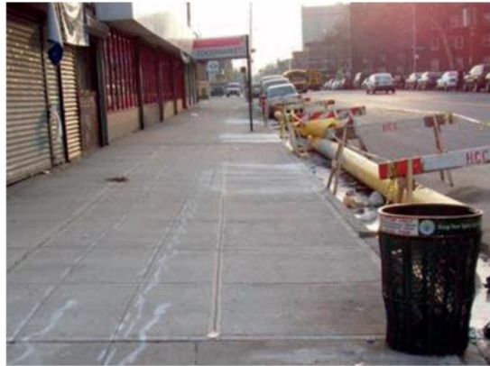
Commercial Corridor: Pre-Construction
