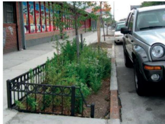
Commercial Corridor: Post-Construction Enhanced Tree Pit
