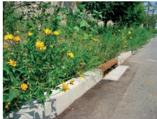
Low Density Residential Street: Post-Construction Infiltration Swale
