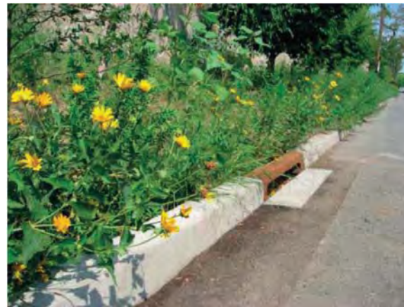
Low Density Residential Street: Post-Construction Infiltration Swale Source: NYC Green Infrastructure Plan
