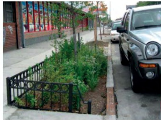
Commercial Corridor: Post-Construction Enhanced Tree Pit
