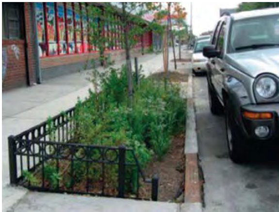
Commercial Corridor: Post-Construction Enhanced Tree Pit Source: NYC Green Infrastructure Plan
