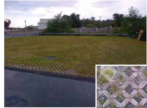
Existing grass-crete treatment used in the City of Glen Cove.
