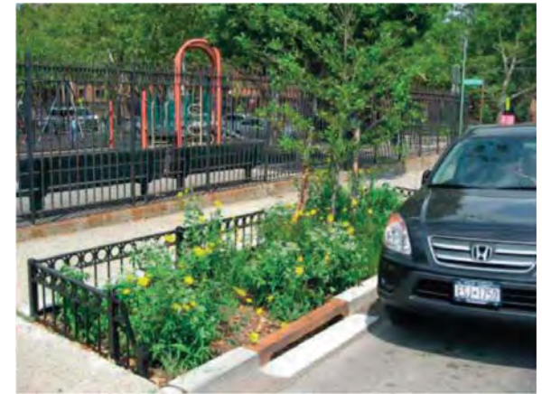
Low Density Residential Street: Post-Construction Enhanced Tree Pit Source: NYC Green Infrastructure Plan
