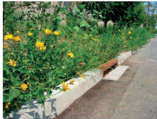
Low Density Residential Street: Post-Construction Infiltration Swale
