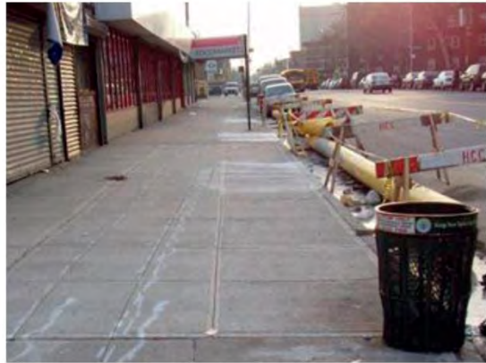
Commercial Corridor: Pre-Construction
