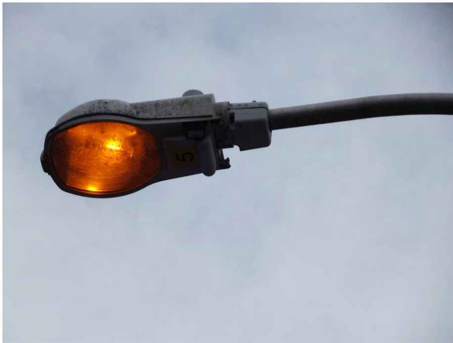
Existing Street Light on Stanco Street
