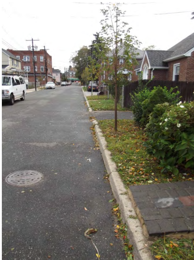
Discontinuous sidewalks on Carney Street looking west toward Hazel Street
