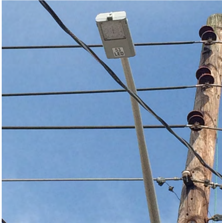
An existing LED street light fixture on Hazel Street
