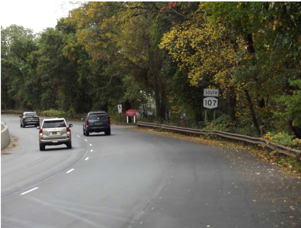
Existing entrance to the Glen Cove Child Care Center Markings are temporary due to recent resurfacing
