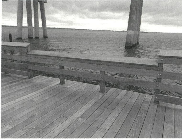
Photo 1. Example of ADA compliant railing at the Old Ponquogue Bridge in Hampton Bays. LKMA designed and performed construction inspection services for this project.
